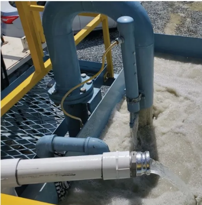
The Settler/Clarifier System can recycle thousands of gallons of water per minute and is closed loop.
